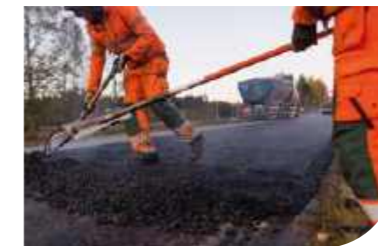
Construction materials and asphalt
